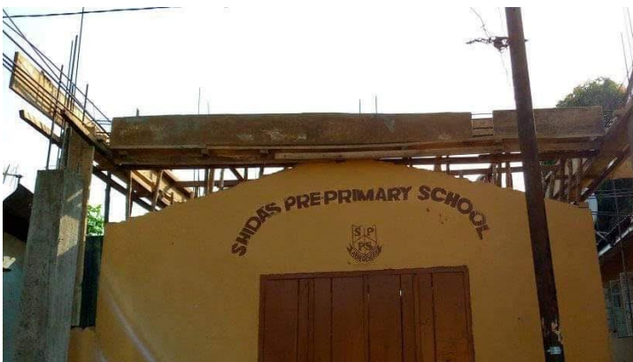
Shida today showing the building work on the second storey. Work has been slowed by Covid and the very high inflation rate in Sierra Leone which has increased costs.
